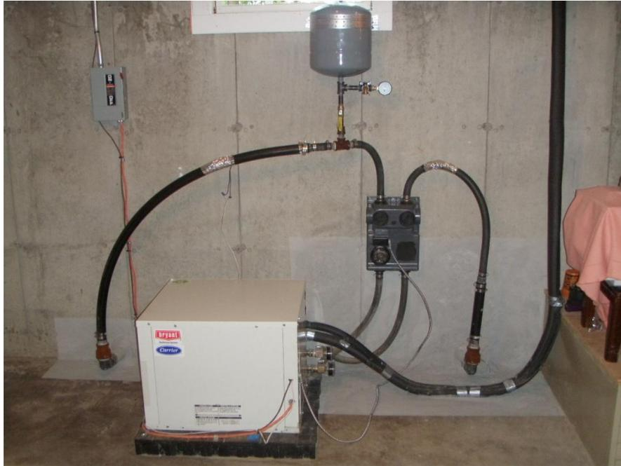
*The buried plastic pipes enter and leave through the basement concrete wall as shown to bring warm water to the Tavino ground source heat pump in winter, and cool water to it in summer.*
